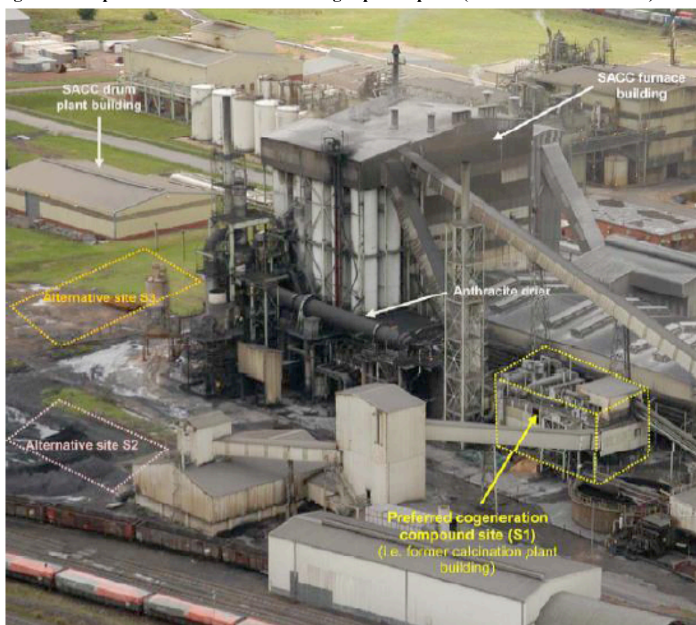
Figure 4: Proposed locations for the waste gas power plant (Source: EIA document)
